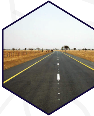
40' WIDE ENTRANCE ROAD
